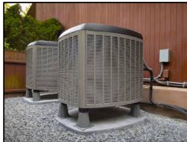
Air Source Heat Pump
